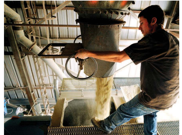
The state's only dedicated organic grain mill was built in 1963 on a 2-acre plot in Auburn, Maine, is right next to the railroad tracks. With its loading and weighing station and 10 storage tanks, the co-op is well positioned to grow. Photo by Daryn Slover/Lewiston Sun-Journal. See story 5/15/10 by Lindsay Tice.
