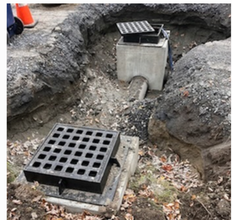
Catch basins installed in the middle of Homestead Acres' roadway.
